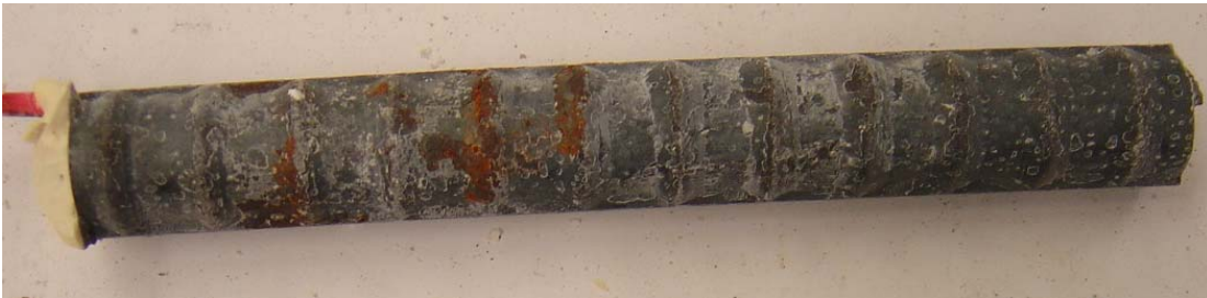
Figure 3.16 – Macrocell Test. Conventional steel from anode specimen (M-Conv.-RH35-6) showing slightly corrosion products at week 25.
