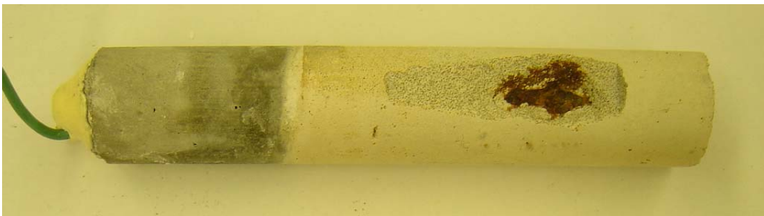
Figure 3.14 – Macrocell Test. Anode specimen (M-Conv.-NO45-2) with conventional steel showing spalled mortar cover at week 15.
