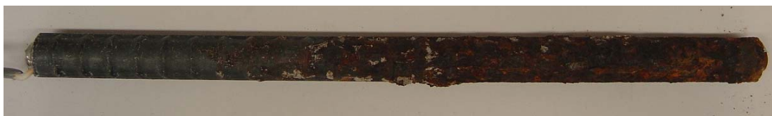
Figure 3.41 – ASTM G109 Test. Conventional steel from bottom mat of the specimen (G-N4-Conv.-6) showing severe corrosion at week 174.
