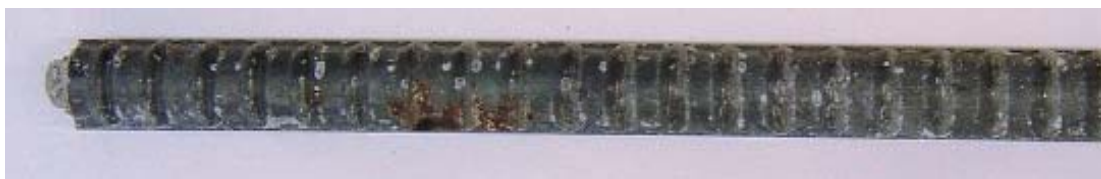
Figure 3.139 – Typical corrosion at initiation on conventional steel.
